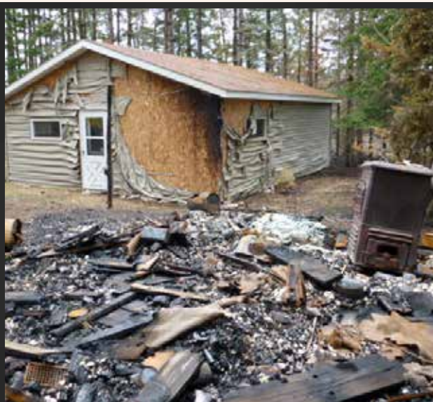
When buildings are too close together the ignition of one can cause neighboring buildings to be damaged or destroyed.
