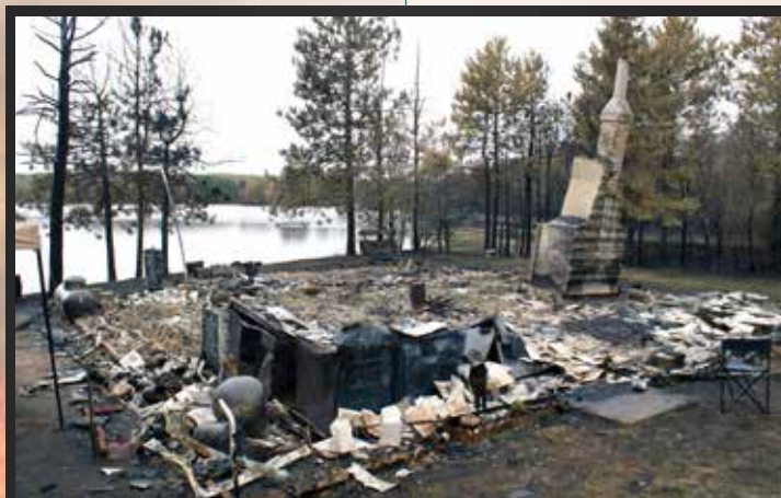
Homes too close to the surrounding vegetation are vulnerable during a wildfire.
