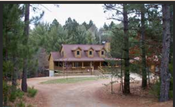
Wildfire risk factors around this home include sandy soils and dense vegetation, especially the pine trees and their fallen needles.
