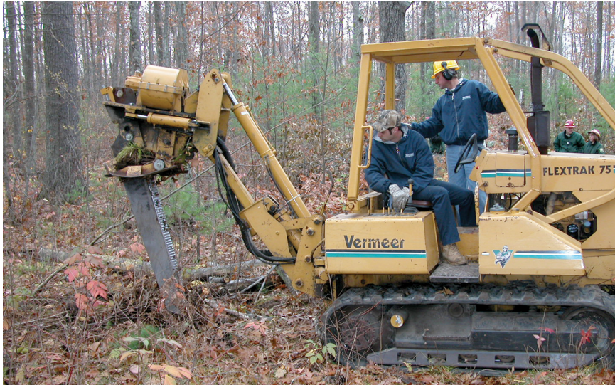
When done correctly, physical root severing is an effective method to stop below-ground spread of oak wilt. Linda Williams, DNR
