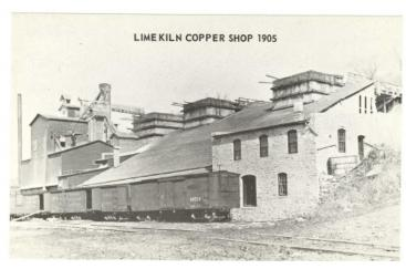
Escarpment. Chemically, limestone is largely calcium carbonate and lime is calcium oxide. Crushed limestone was heated to break down the calcium carbonate, leaving lime as the end product.
