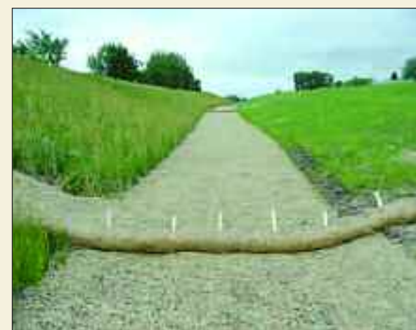
ABOVE: Temporary ditch check with sediment log
