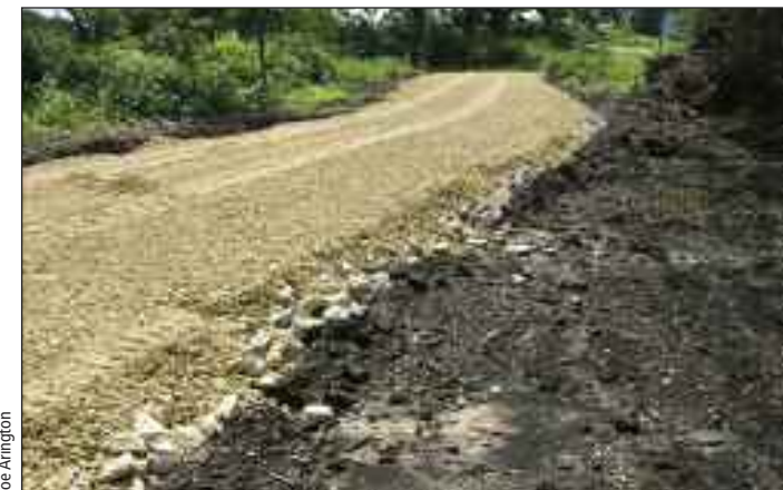
LEFT: Permanent wetland crossing after construction with breaker run and gravel
