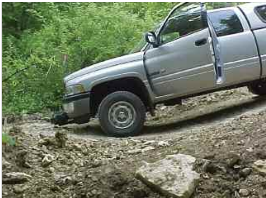
ABOVE: Construct broad-based dips shallow enough to accommodate expected vehicles.
