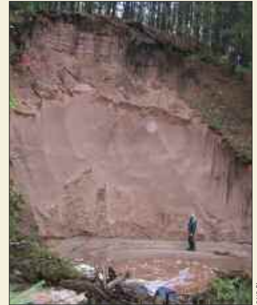
RIGHT: The streambanks in this area of the state are extremely susceptible to in-stream erosion.
