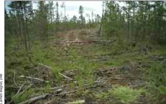
LEFT: Temporary wetland crossing on frozen ground using slash
