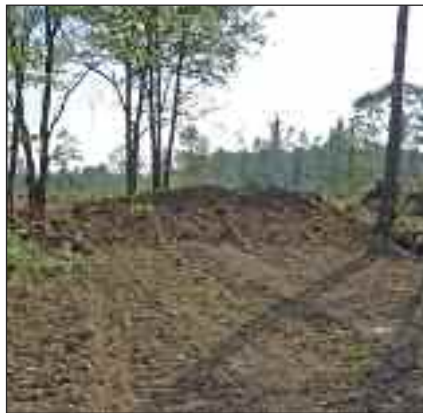
ABOVE: Berms are effective when frequent access is not required
