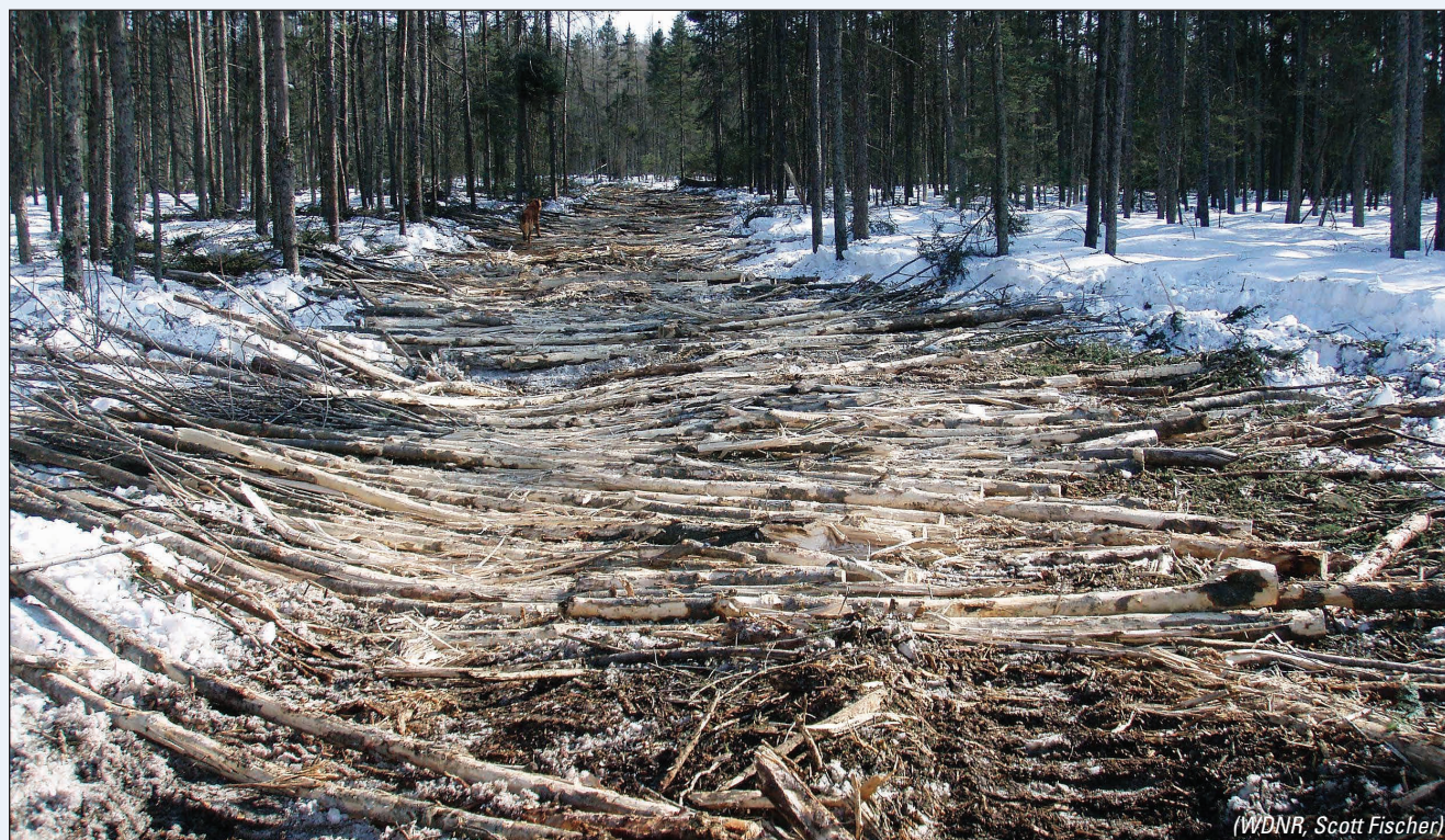
Figure 12-27: By using log corduroy at this timber harvest, the loggers were able to safely extend their operating season without damaging the wetland.
