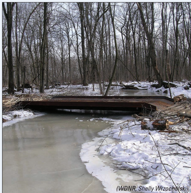
Figure 12-13: This temporary bridge provides access for forest management activities when a permanent crossing is not needed.
