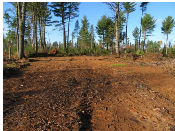
Figure 24. Traditional type landing includes a large turn-a-round build into the forest road system.
