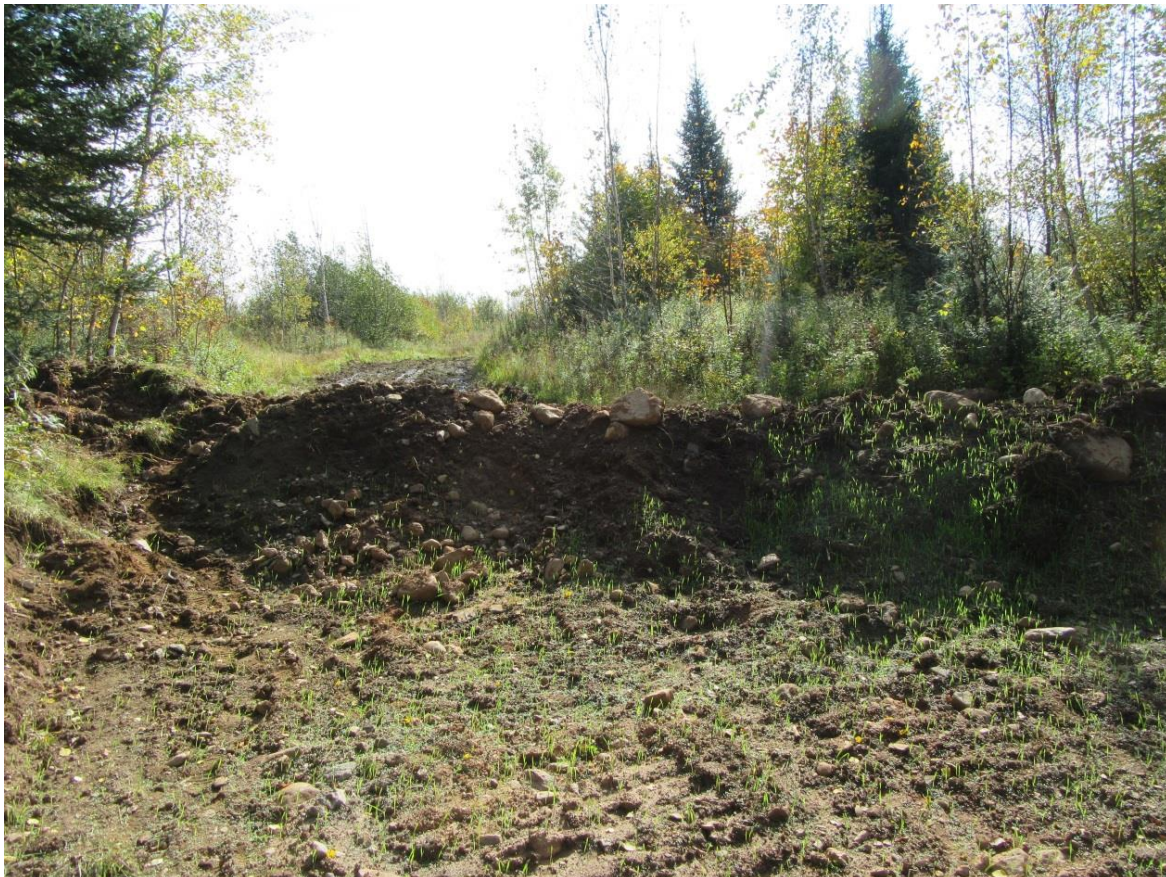
Figure 7. A forest road that has been blocked to keep traffic out by an earthen berm. The harvest on this forest road system was seasonally restricted (winter). Barriers are the best way to stop soil disturbance that could occur if sensitive sites are exposed to traffic after the harvest is completed.
