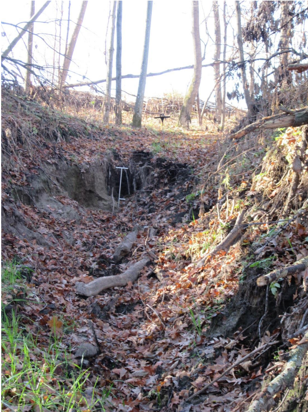
Figure 21. The deepest gully found during the study. It was discovered on state property in the driftless area. The location of the road is at the bottom of two slopes. Since there was no drainage structures present to control the water magnitude or velocity, the water naturally concentrated in this area, and created this deep gully which engulfed almost the entire width of this forest road.
