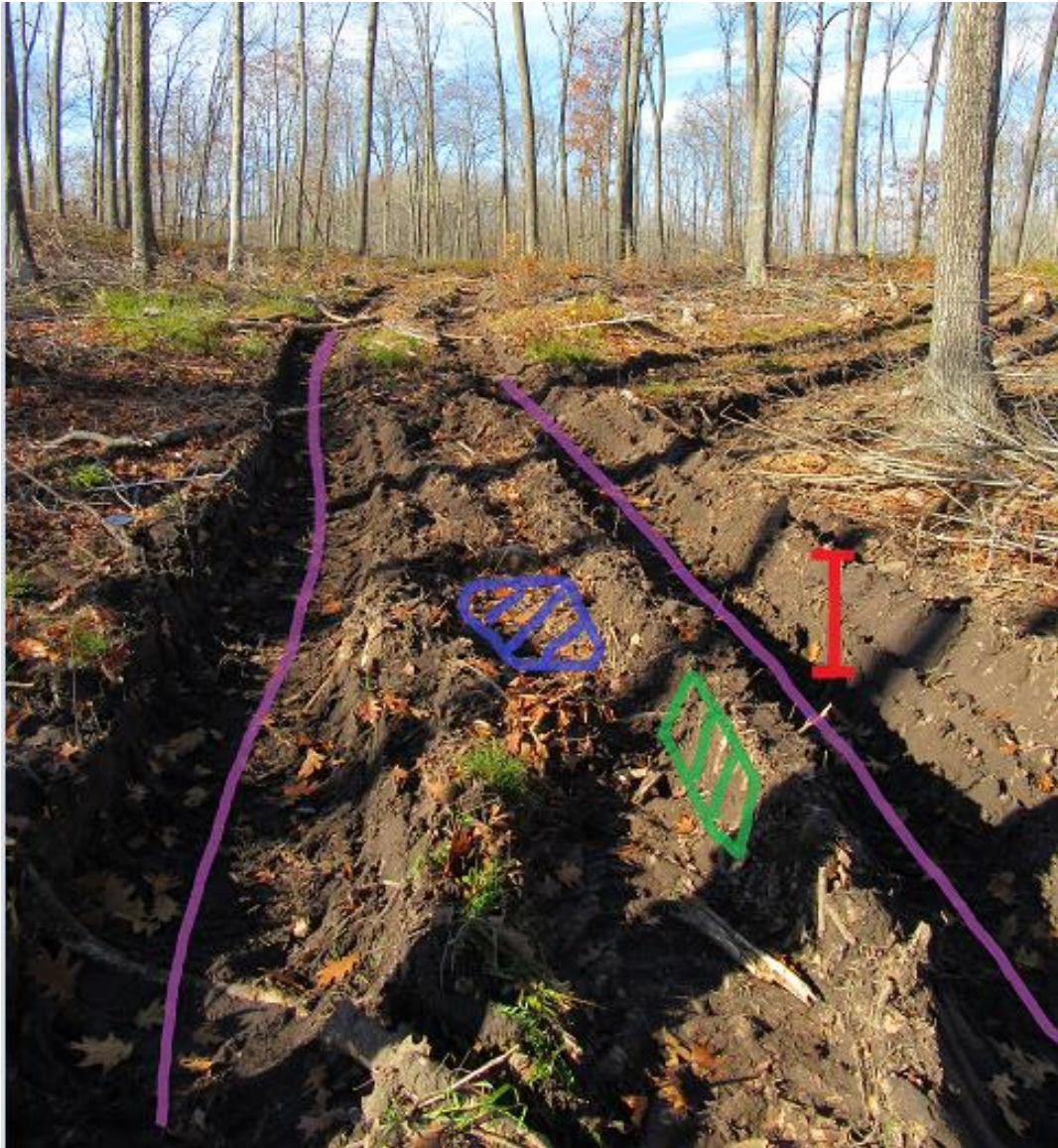
Figure 8. Purple lines represent the distance where the rut is over 6" deep to the original ground surface (represented in blue). The red line represents the maximum depth to the top of the soil. Green lines outline soil which was pushed out of the ruts and is above the original ground surface.
