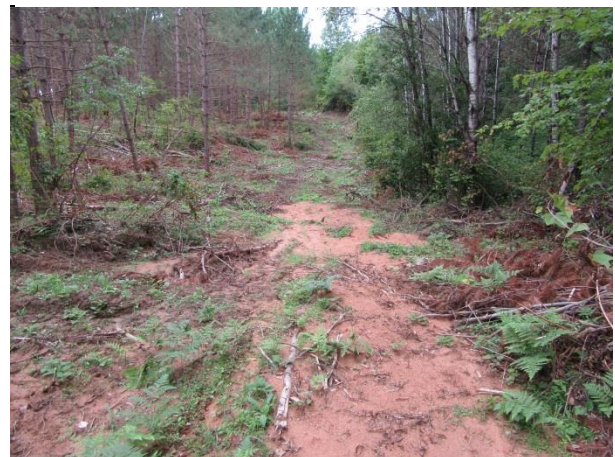
Figure 3. Displaced sediment from the gullies on the forest road shown in figure 2. This sediment will make it more challenging for the road to re-vegetate and become stable.
