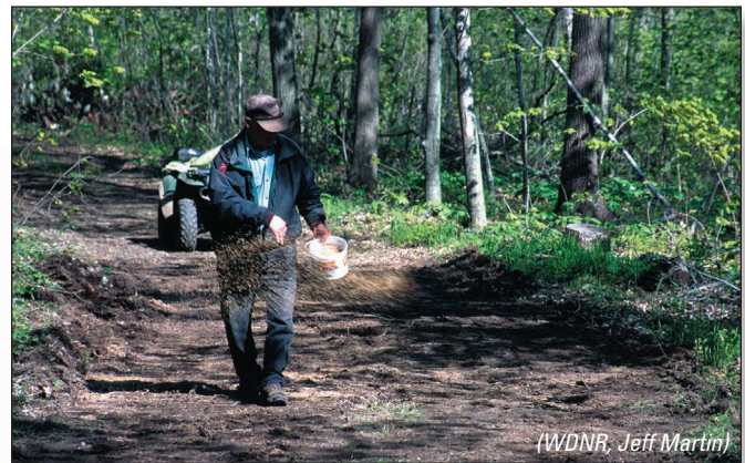
Figure 16-20: Seeding can be as easy as spreading grass seed by hand as this landowner is doing on his freshly-graded woods road. Use non-invasive species and certified weed-free seed.
