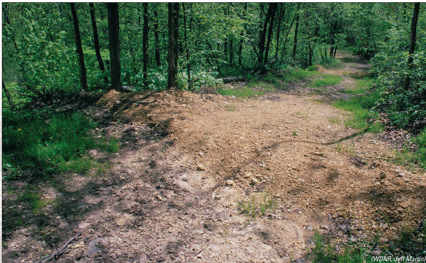
Figure 12-17: This waterbar, placed at the proper angle to the road, will intercept runoff water and direct it into the adjoining vegetation.
