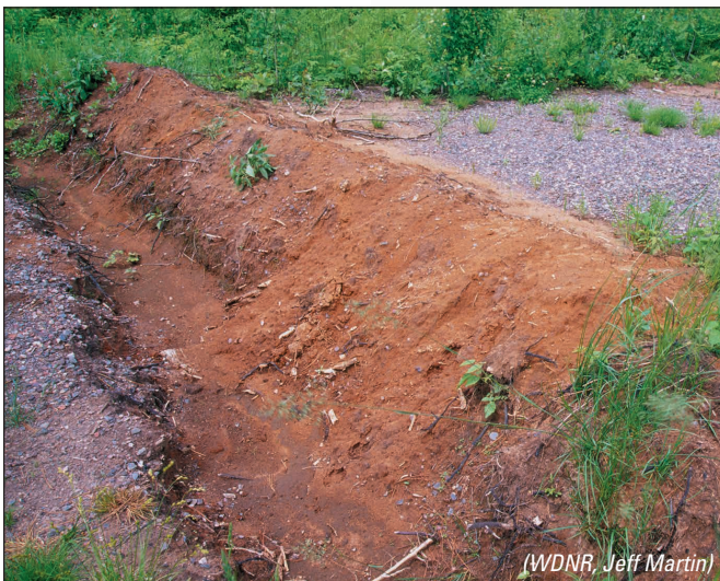
Figure 11-3: At the end of a forest operation, a simple earthen traffic barrier may be satisfactory for preventing unwanted vehicle traffic.
