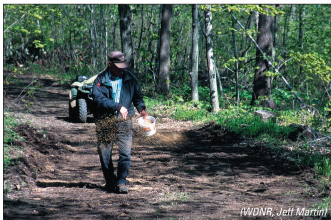
Figure 12-1: Seeding can be as easy as spreading grass seed by hand as this landowner is doing on his freshly-graded woods road. Use non-invasive species and certified weed-free seed.
