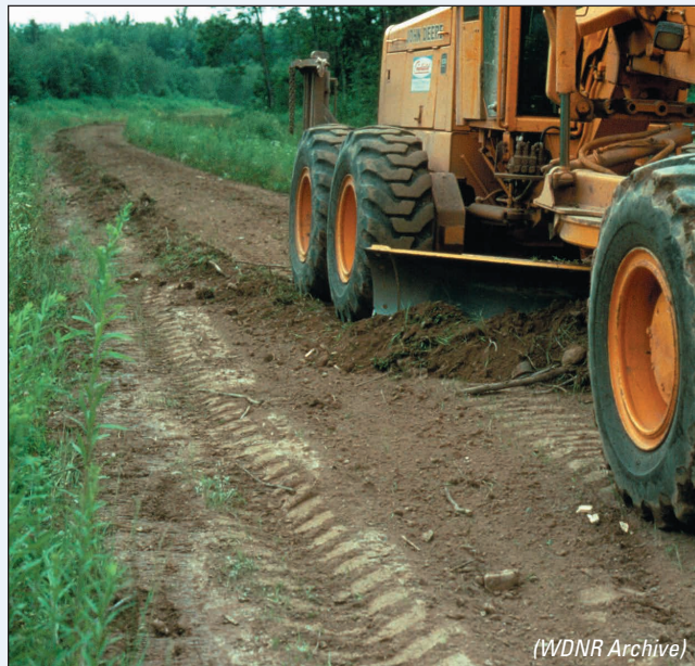
Figure 12-28: Maintaining woods roads helps prevent erosion. This grader is shaping the road surface so that water runs off properly.
