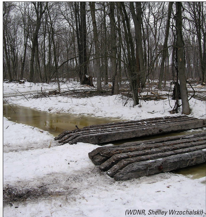
Figure 5-3: Temporary stream crossings can provide access to areas not needing permanent access, while allowing the timber harvest, and greatly reducing the potential impacts of the stream crossing.
